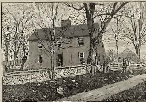
HOUSE BUILT BY THOMAS HAWLEY AT STEPNEY, CT., IN 1755.
